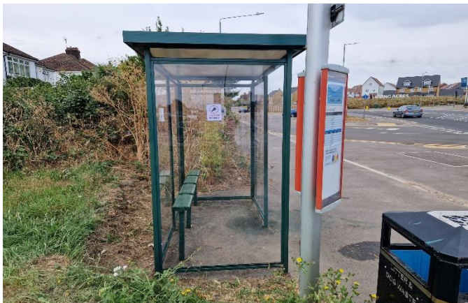
Replacement Panels installed
